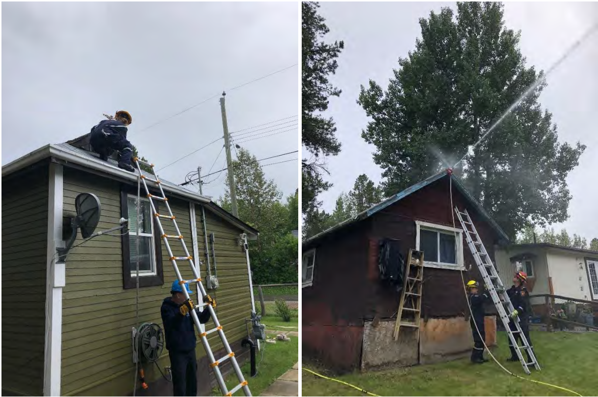
Installing sprinklers on a house in Robb.
