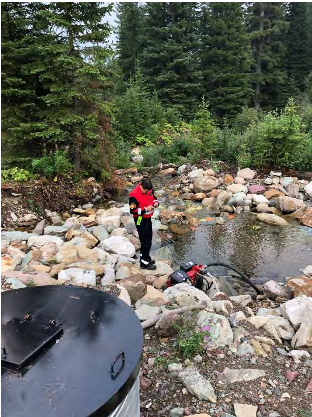
Checking a pump site in Castle Mountain.
